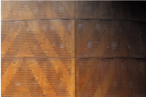
Cook Landing Tukutuku Panels 4. Perforated metal panels to create pattern and texture.
