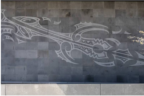
Tūhura 2. Patterns etched onto concrete or paving
