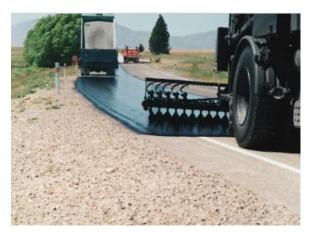
Image from NZTA - Chipsealing in New Zealand
