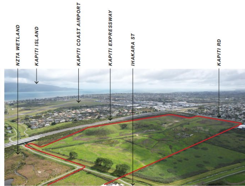
Fig 4. Aerial view from the South looking North
