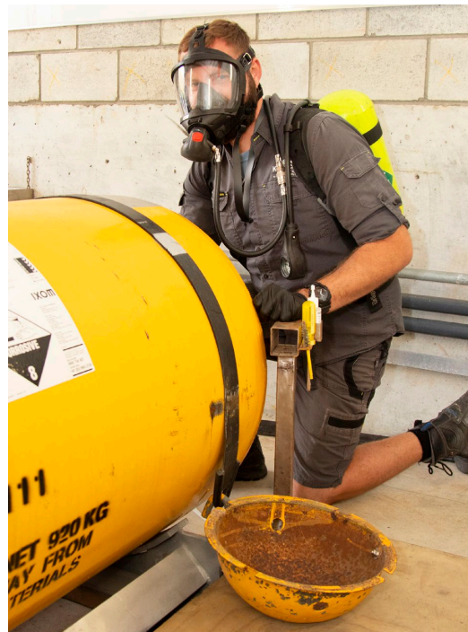
Worker using a self-contained breathing apparatus to replace an empty 920kg 100% concentration chlorine gas cylinder. As per the safe operating procedure.
