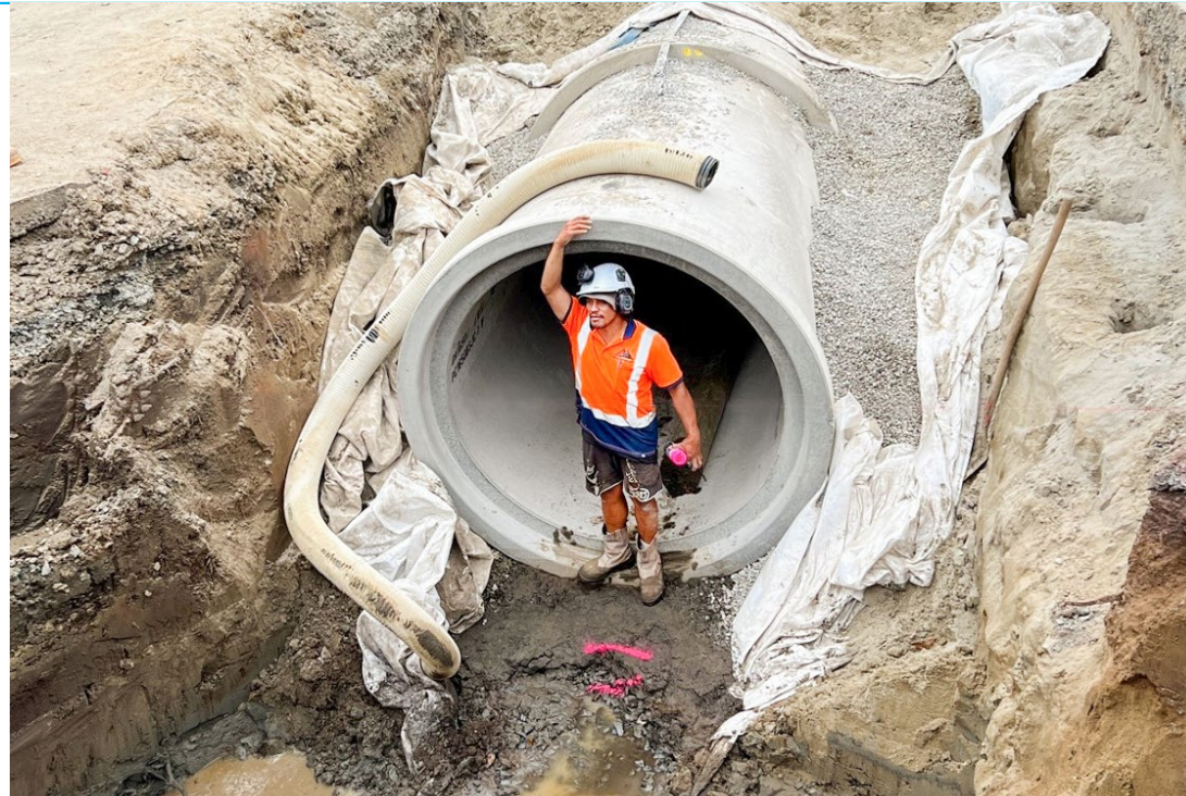
Installation of 800 metres of large diameter stormwater pipe from Iver Trask Place to Amohia Street to reduce flooding issues.
