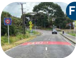
New Threshold treatment, e.g., 30/50
