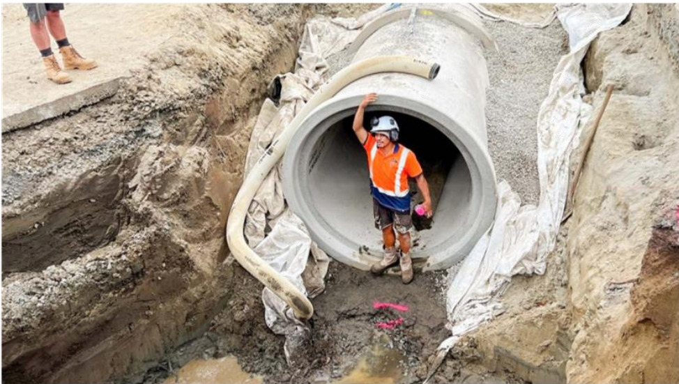
Amohia stormwater pipe installation.
