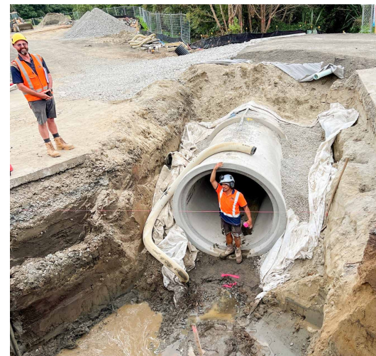
Installation of 800 metres of large diameter stormwater pipe from Iver Trask Place to Amohia Street to reduce flooding issues.
