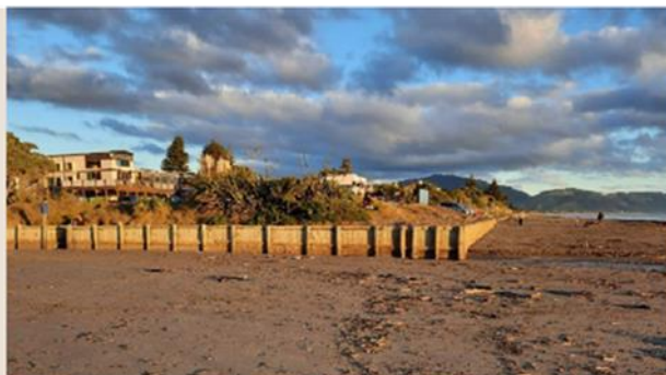
We rebuilt the retaining wall at the mouth of Wharemauku Stream at Raumati Beach to manage stormwater and sea-level rise.
